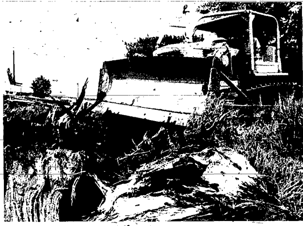
Cleaning Up Clearing of the Gibson store site began this week by Carlson Construction Co. Construction of the 27,000-square-foot building is to begin soon.
